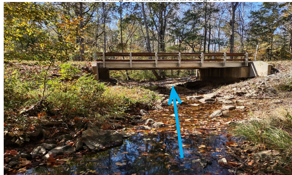
View Looking Downstream from Bridge 286
