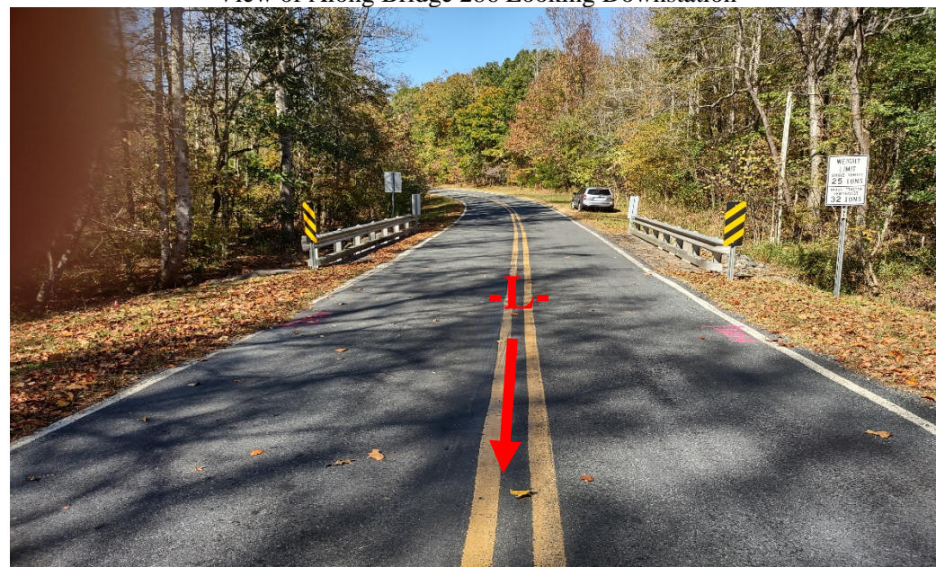
View of Along Bridge 286 Looking Downstation
