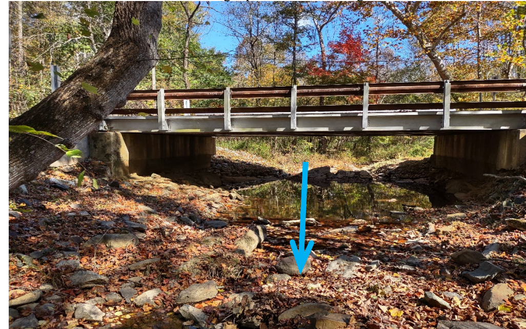
View Looking Upstream from Bridge 286
