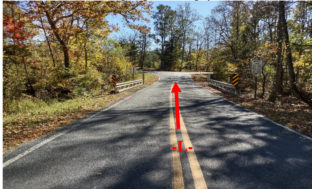
View Along Bridge 286 Looking Upstation
